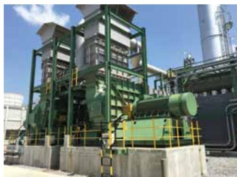
Two Design 5500 Forced Draft Fans, size 7678, Backward Curved w/Flue Gas Recirculation, designed to handle 115,753 ACFM & 49"wg for a Boiler application in Thailand.
