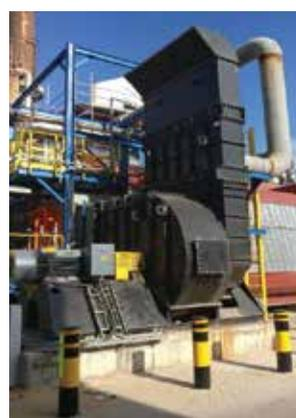
Heavy Duty Custom FD Fan w/FGR used in boiler application at a refinery.
