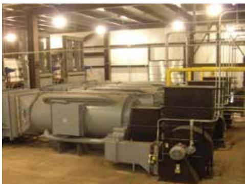
Burner installation utilizing three size 2700 Arrangement 4 Packaged Forced Draft Fans.
