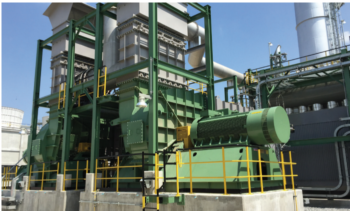
These two Design 5500 Forced Draft Fans are size 7678, Backward Curved w/Flue Gas Recirculation and are designed to handle 115,753 ACFM & 49" w/g for a Boiler application in Thailand.
