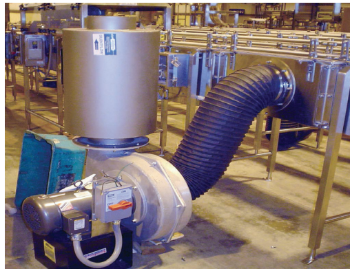
Cast Aluminum Pressure Blower installed on a vacuum conveyor.
